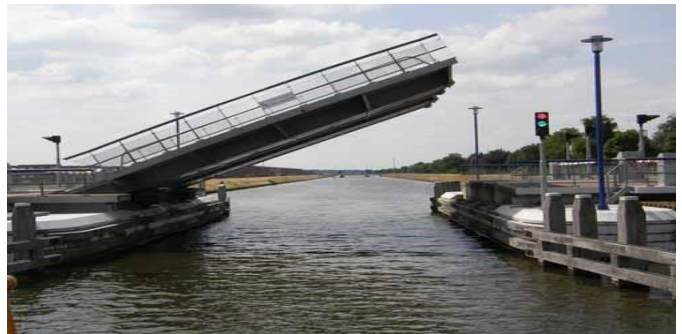
Sluices Rogat Bridge
